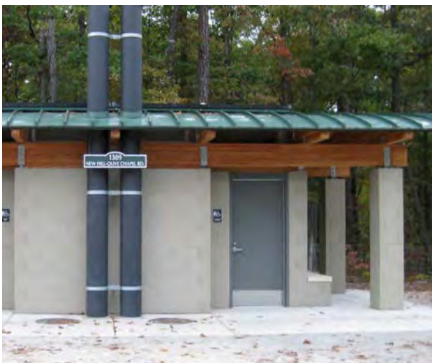
Composting restroom at the current southern end of the American Tobacco Trail in Wake County.
