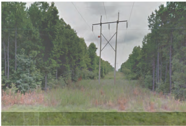
Existing conditions along utility corridor
