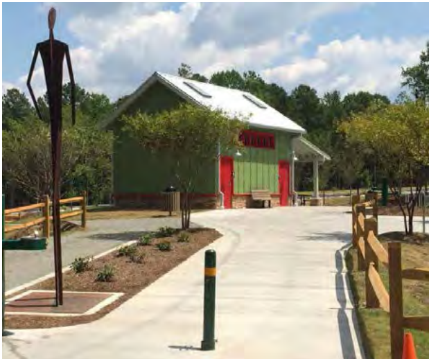
The New Hope Church Road Trailhead Park in northwest Cary.
