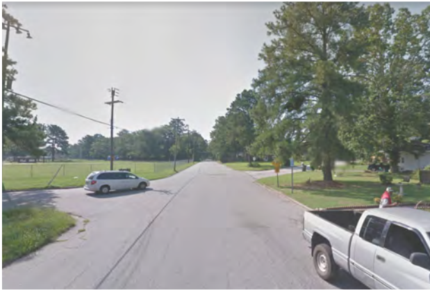
Existing Conditions at Avondale and Ridgecrest
